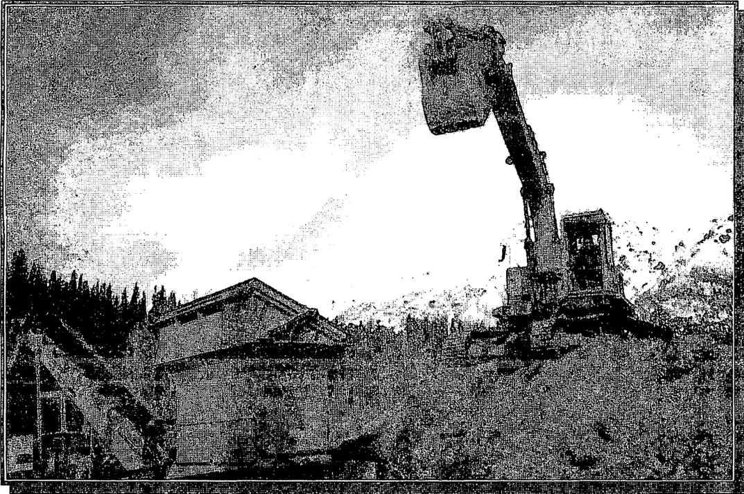
This is the gravel screening plant Miller-Bock General Contractors set up near the Lakina River, about a mile west of Long Lake. First the large rocks are removed, then the fine dirt and sand. The final product is then trucked to the repair site, the area along the lake where part of the road fell off into the water in 1994.
