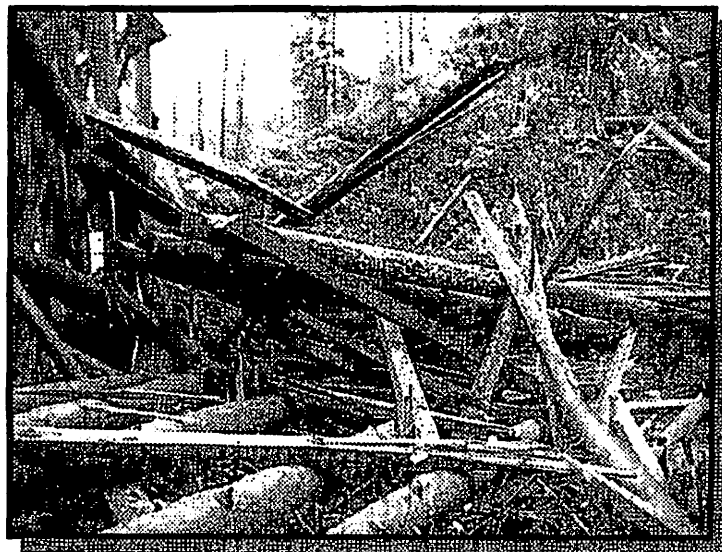
TRESTLE AT HALEY CREEK.
