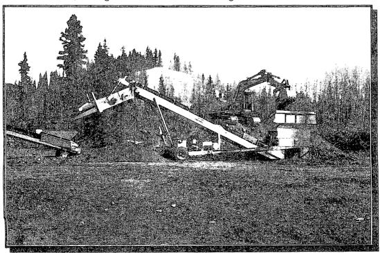
The hillside was cut back away from the lake, then a deep trench dug the length of the repair area, then filled with gravel from the screening plant. Removed material was hauled several miles to the east end of the lake, so that no dirt would get into the lake itself.
